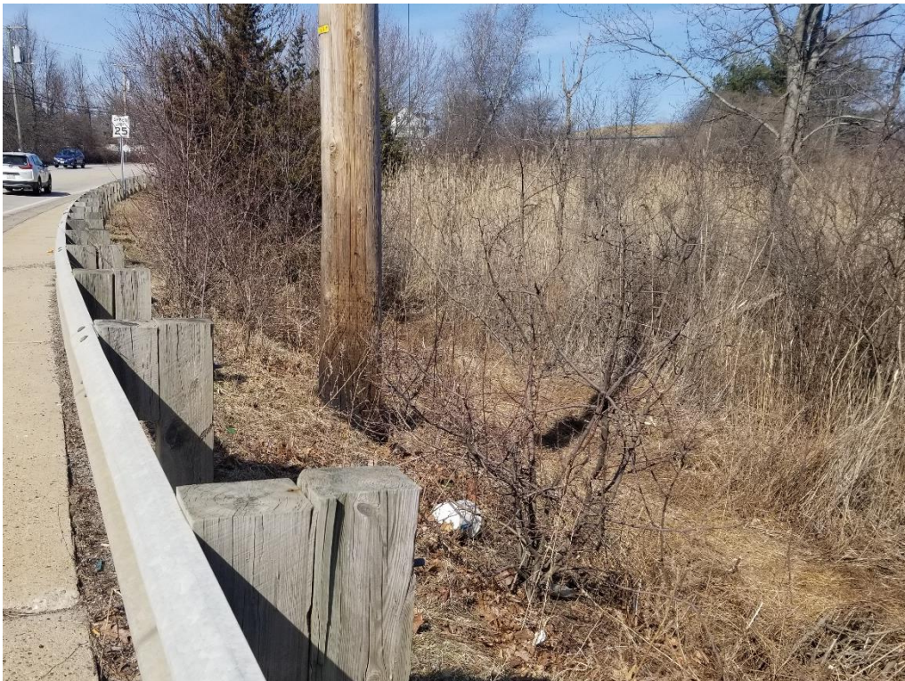
Photo 2: Wetland B (T.I.A. 9; P.I.A. 10), facing north along Peverly Hill Road (03/13/2024)
